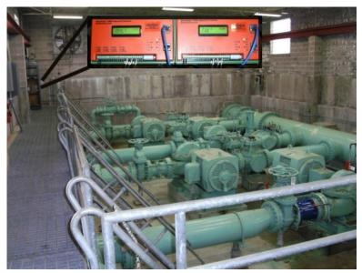
Photo of the 50MGD Pump Station. Four Sensus Turbo Meters (16 Inch), which were outfitted with ICE<sup>®</sup> registers, are now monitored by two EtherMeters<sup>TM</sup>. The meters (not shown) are located in a below-grade vault several hundred feet from the pump station. The industrial communication protocol used is MODBUS<sup>®</sup> TCP.
