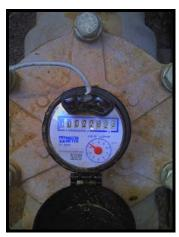
6 Inch MMT Turbo Meter, Installed At One Of The Air Force Base's Well Stations.
