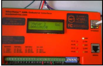
EtherMeter Connected to The 6 Inch MMT Turbo Meter. Communications To The Base Energy Management System Is Via MODBUS/TCP. Note The Perfect Agreement Between The AccuLinx Register and the EtherMeter.
